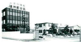
浜松市葵町の遠州軽合金(株) En-Shuu Kei-go-kin (light alloy) Co., Ltd at Aoi-cho, Hamamatsu City.
